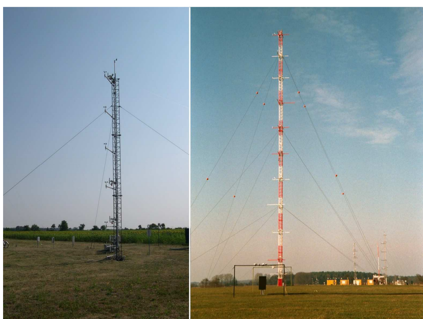
Figure 4: A 10-m mast (left) and a 99-m tower (right) deliver wind data with over 98% availability.
